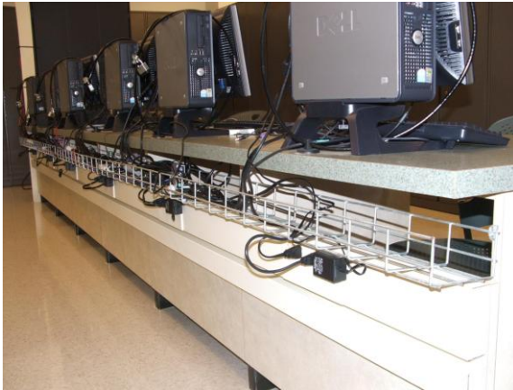
Illustration 3: View of a row of workstations, showing the wire trough for laying network cabling.
